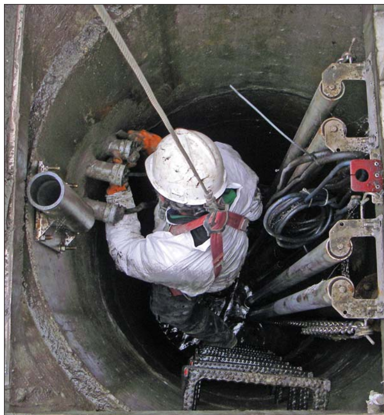
A Miksis Services worker makes a confined-space entry down a manhole to prepare a pipe-bursting pull. (Photo courtesy of Miksis Services Inc.)
