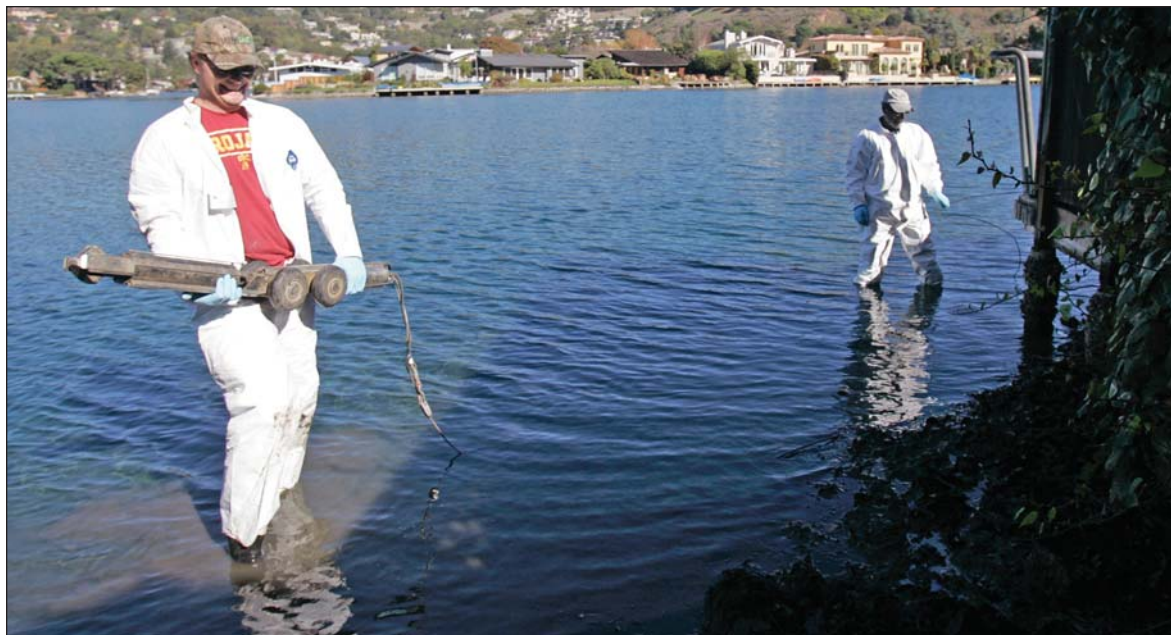
Steve Miksis, left, and Sal Galindo carry an Omni Eye-2 camera from RS Technical Services Inc. while preparing to send it into a sewer line. (Photo by Chad Surmick)
