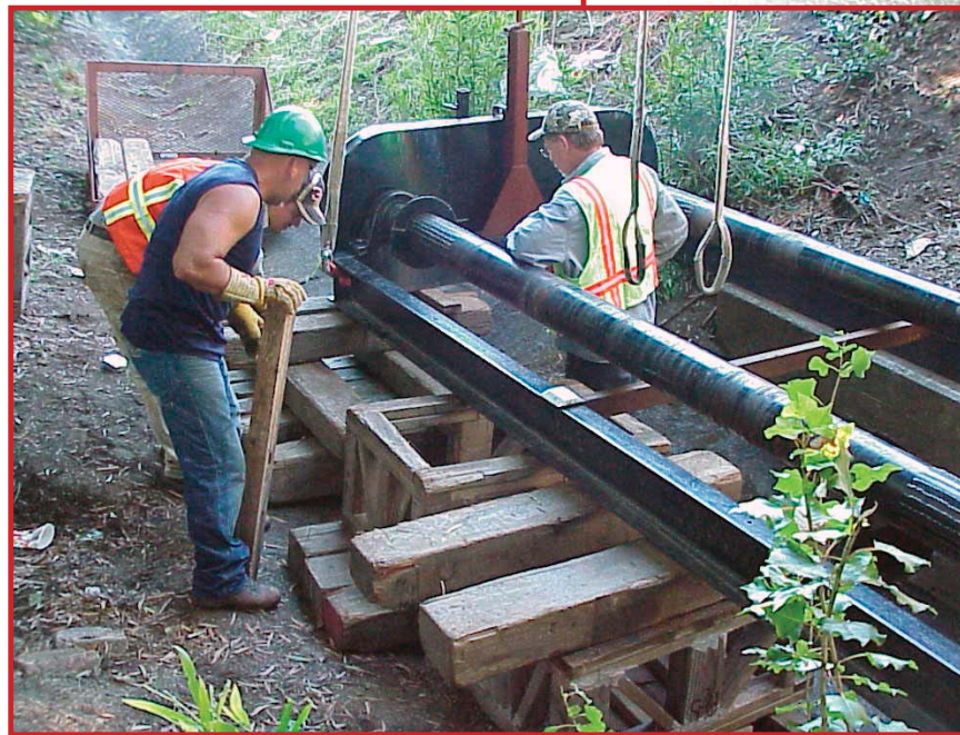
UltraLiner representative Lee Trotter (right) oversees building the cribbing and special rollers for launching the liner.
