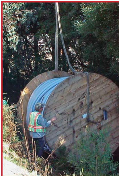
The folded UltraLiner and its 8-foot-tall wooden spool weighed a combined 16,000 pounds.
