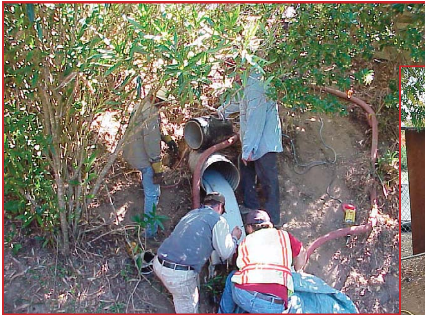
Above, feeding the liner into the culvert. At right, an old 30,000-pound logging winch was crucial to completing the pull.
