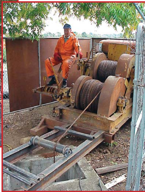
Above, feeding the liner into the culvert. At right, an old 30,000-pound logging winch was crucial to completing the pull.
